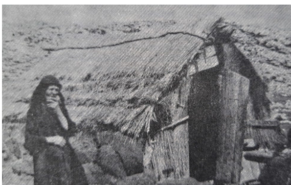
Figure 7. „Mlikar“ wooden structure with turf cladding (Mihić, 1985)
